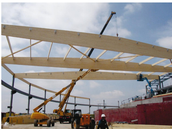
Beginning of the roof structure of the experiment area of SOLEIL.
