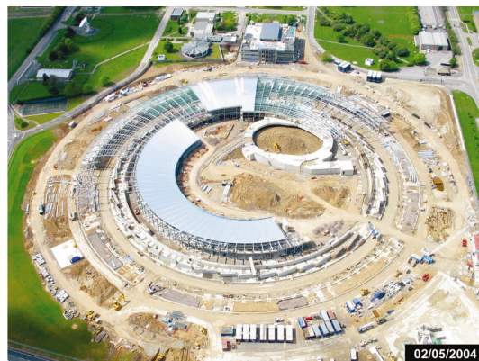
Bird's-eye view of the construction site.
