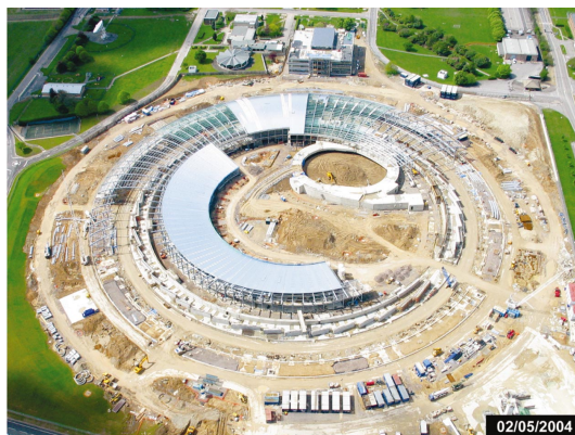
Bird's-eye view of the construction site.
