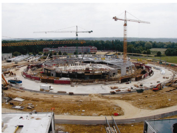
General view of the SOLEIL building site on 3 June 2004.
