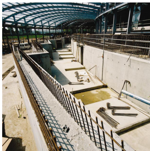
Storage-ring tunnel and pre-cast roof.
