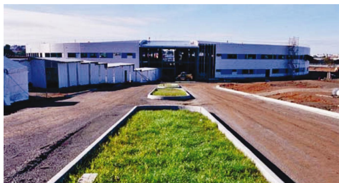
Outer shell of the Australian synchrotron building.
