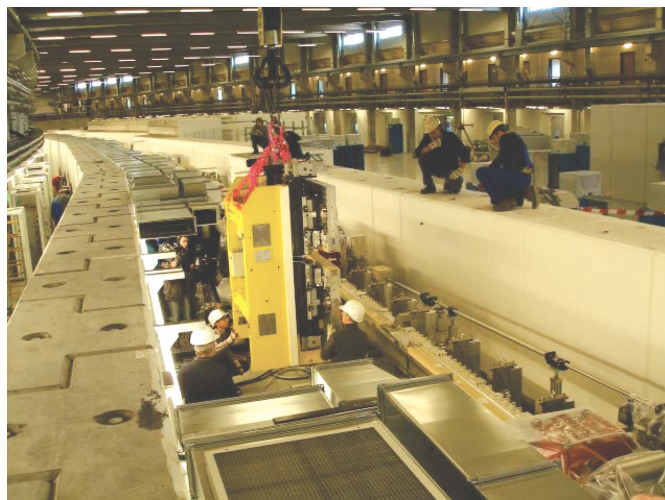
The 5.8 ton PETRA III undulator is lifted into place.
