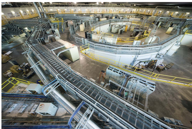
Inside view of the CLS. (Photograph courtesy of the Canadian Light Source.)
